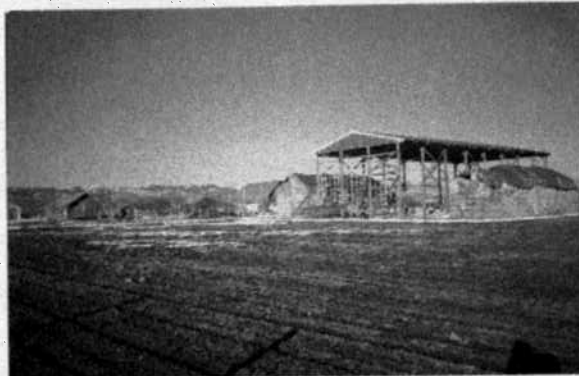
Large open-sided pole buildings have replaced the more traditional barns in the Kittitas Valley timothy landscape.
