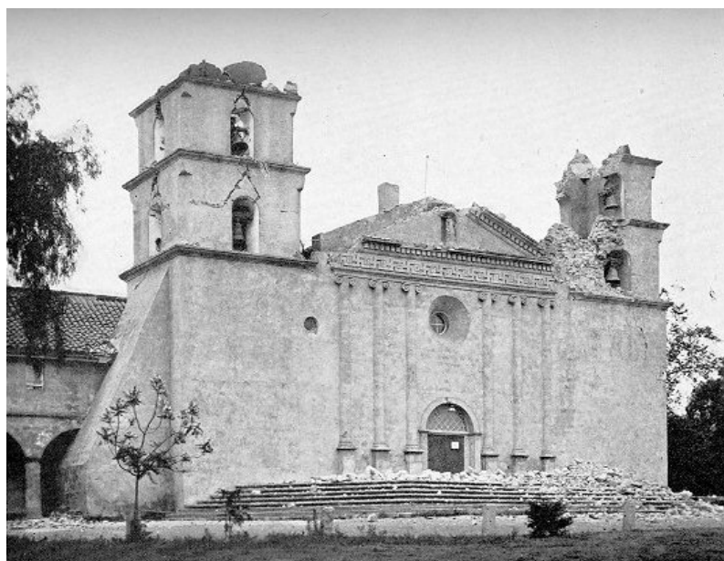
Santa Barbara Mission after the 1925 earthquake. Image from the Santa Barbara Earthquake History Web Page ( http://www.crystal.ucsb.edu/ics/sb_eqs/ ). Image scanned from the Bulletin of the Seismological Society of America , v. 15, Dec., 1925.
