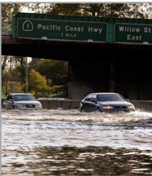
Flooding along the I-710 freeway in Long Beach, California (Kevork Djansezian 2017)
