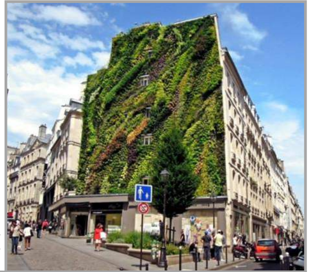
Green wall in Paris, France designed by Patrick Blanc. Example of a built form of green infrastructure.
