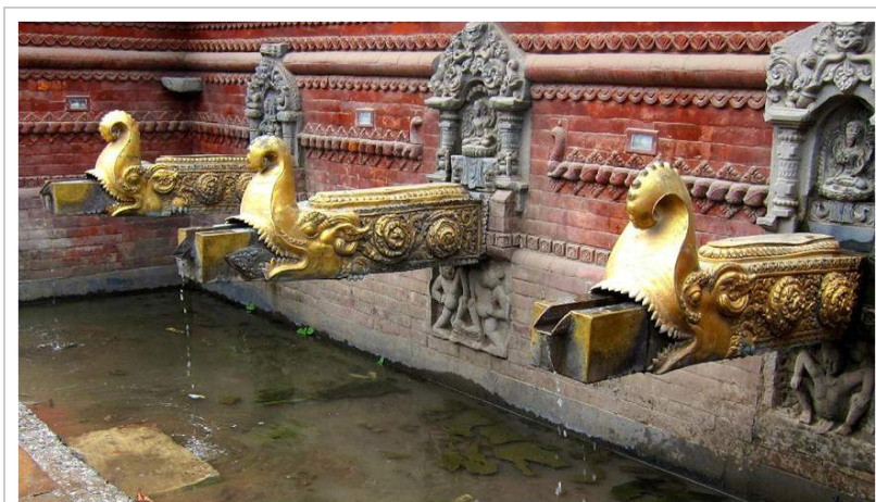
Figure 3: Since the 1990s Sun Dhara Hiti only flows during the monsoon because wells in an industrial estate upstream lower the water table. This has led to protests and unresolved conflicts with the municipal government.
